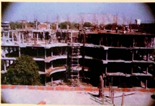
SHYAM ANUKAMPA APARTMENTS (Under Construction)
